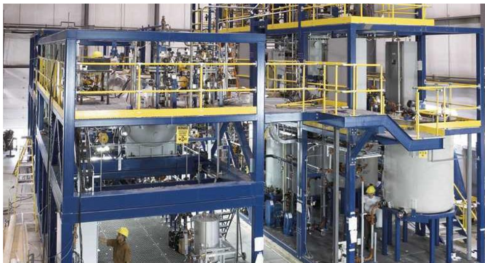
Figure 5. This demonstration-scale hydromet plant designed by Hatch and built by Zeton had thirteen different wetted materials of construction in piping.
