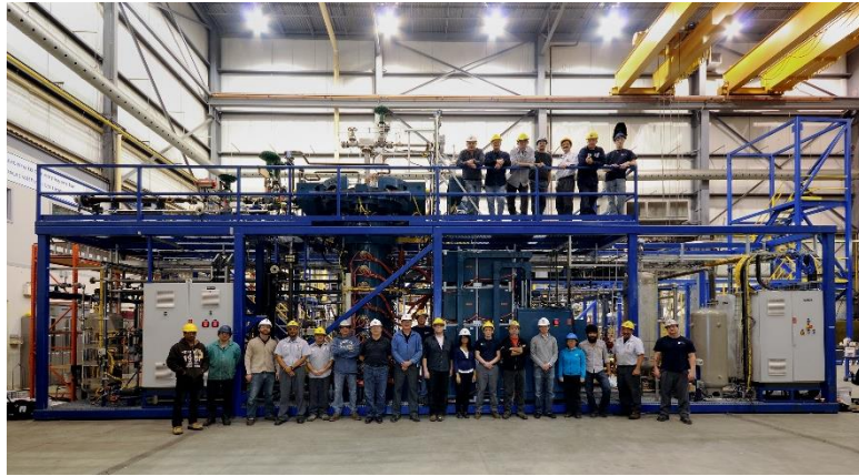
Figure 2. This pilot plant had a reactor with an extremely challenging design point: 2500 psig at 1200 °C.
