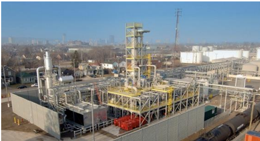
Figure 13. This 60 million litres per year continuous biodiesel production plant was executed by Zeton using our design–build modular approach.
