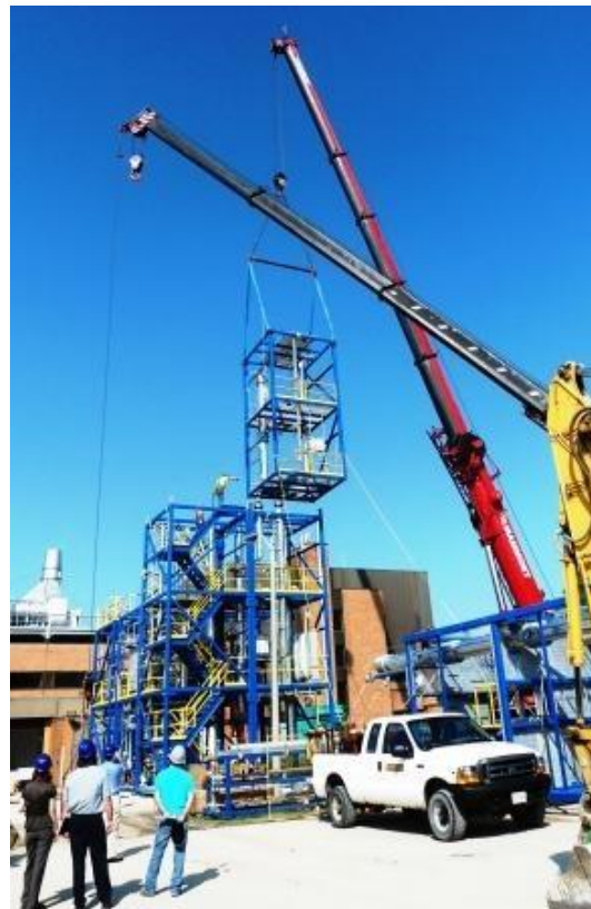
Figure 17. Zeton's pre-engineered vertical and horizontal modules stack together quickly and efficiently.
